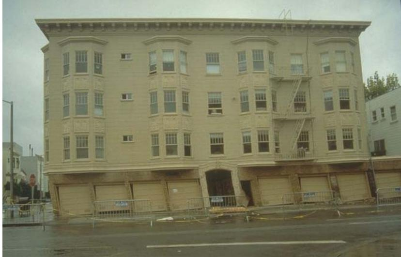
**Figure 1.1.** Multi-unit apartment building that suffered a weak-story failure in the 1989 Loma Prieta earthquake. Note the presence of garage doors at the ground story. (Raymond B. Seed, National Information Service for Earthquake Engineering, University of California, Berkeley)
